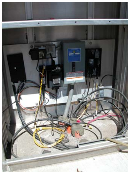
Figure 4.3 – CCTV Cabinet Installation CLOSE-UP OF CABINET INTERIOR
