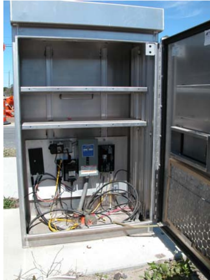
Figure 4.2 – CCTV Cabinet Installation CABINET INTERIOR
