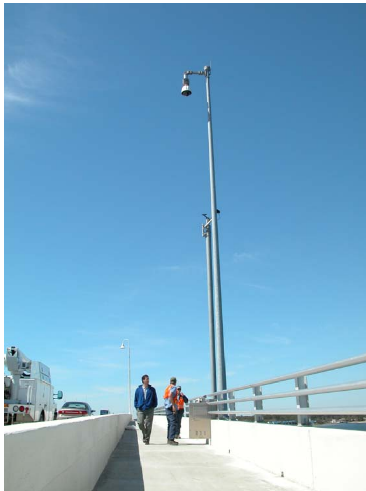
Figure 4.11 – CCTV / RWIS Site on the Hathaway Bridge
