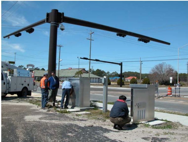
Figure 4.1 – CCTV Location U.S. HIGHWAY 98 – WEST OF HATHAWAY BRIDGE
